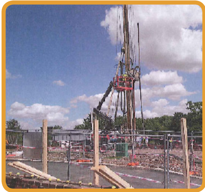
Phase 1A on site
