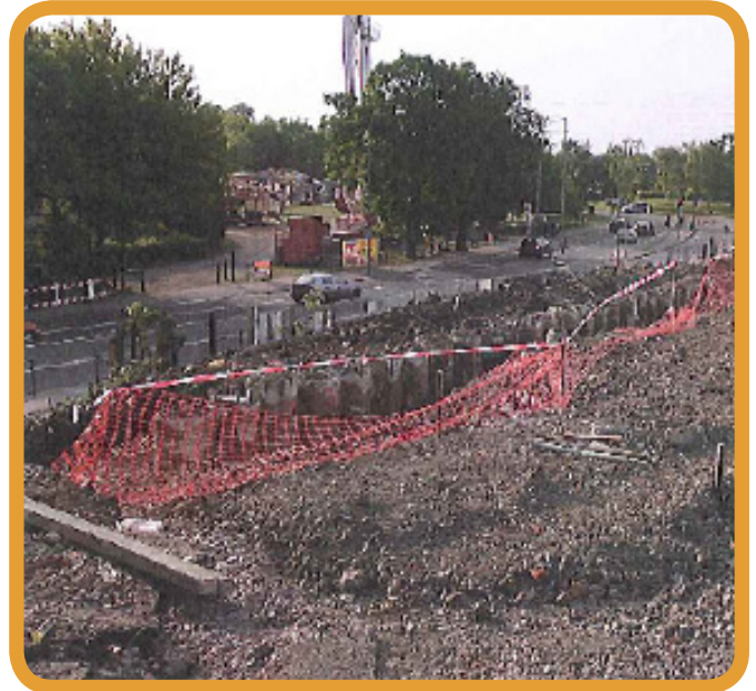
Phase 1B on site
